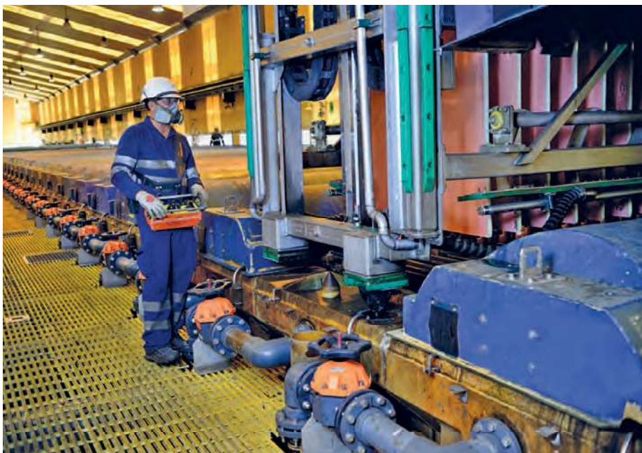
The 144 electrowinning cells – containing 82 cathodes and 83 lead anodes – help produce LME grade copper cathodes weighing around 50 kg each
